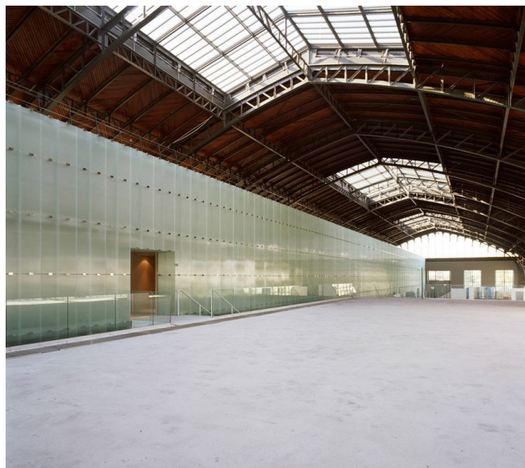
Water Centre SCAU
